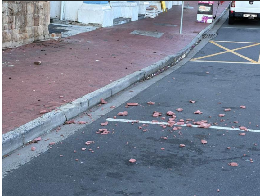
Figure 2. Roof tiles which were dislodged by baboons and subsequently fell on to Simon's Town Main Road.
